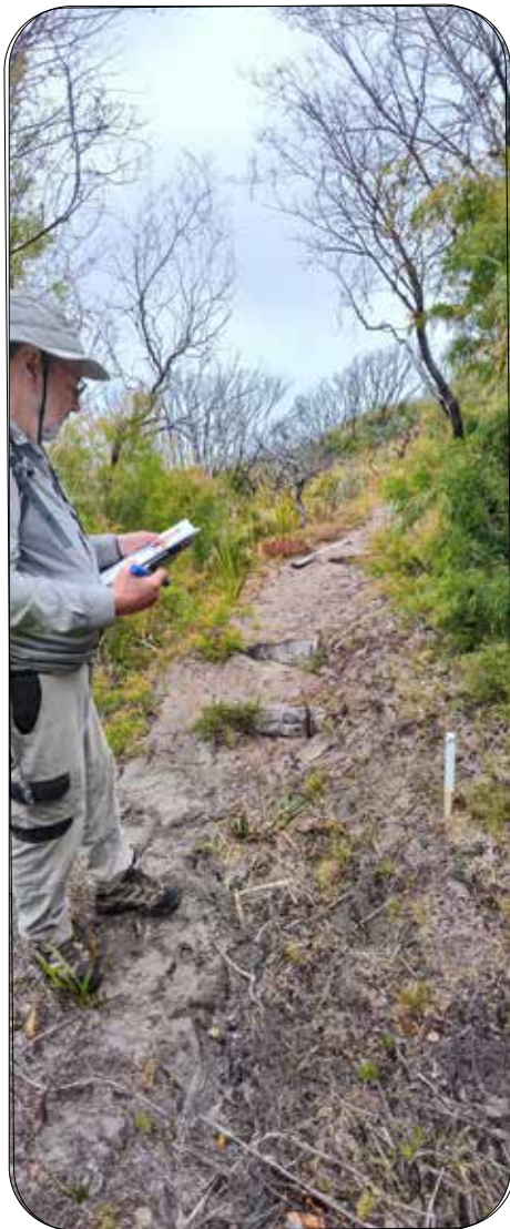
Ross marking start of repair section
