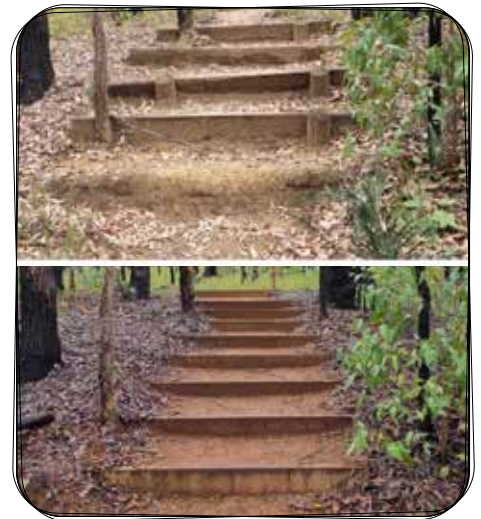
Before/After repair to stairs at Noggerup.
