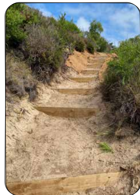
Section of repaired Track
