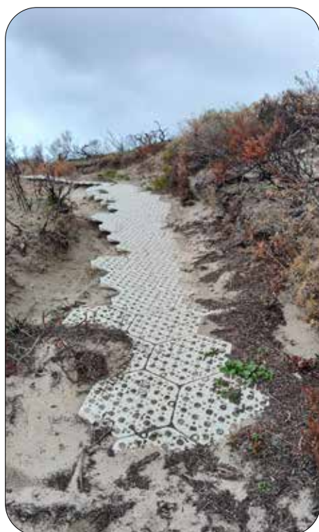
Trial trackpad needing replacement.
