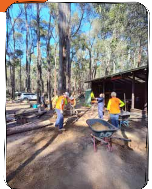
Digging the footings for the shelter extension
