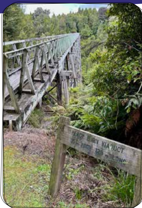
Percy Burn viaduct
