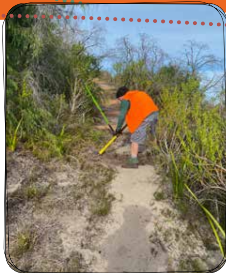
Bill installing a new step.
