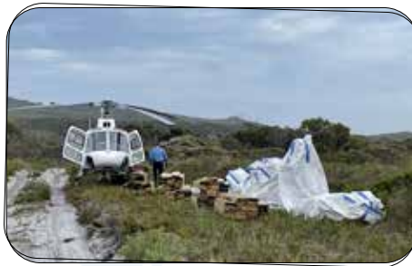
Preparing loads for air-lift.
