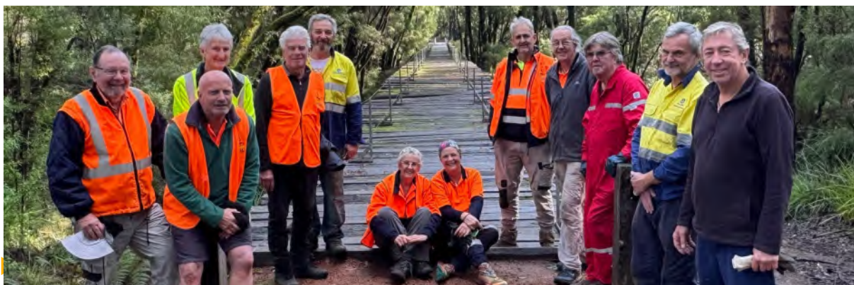
► Support Volunteers celebrate completing their triennial maintenance visit to River Road Bridge.
