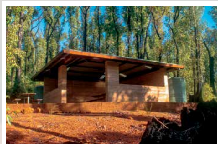
Over the years, timber shelters lost to bushfires have been replaced by rammed earth.
