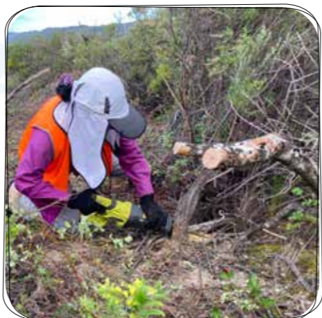
Volunteer using reciprocating saw on the Nullaki realignment
