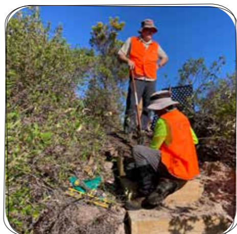
Building box steps on the Nullaki realignment
