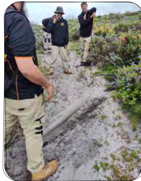
The Binalup Rangers hard at work repairing a waterbar.
