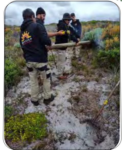
Rangers repair a waterbar.
