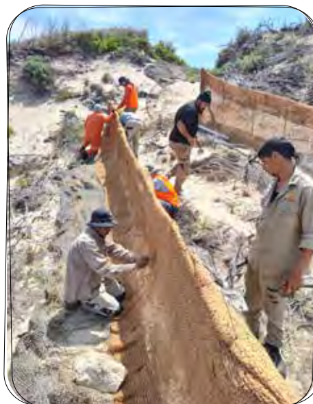
Repairing the wind fences.
