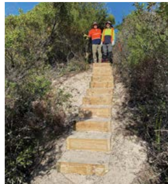
▶ Volunteers constructed steps on the Nullaki Peninsula route
