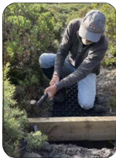
South Coast Stabilisation – John Hosking installing steps.
