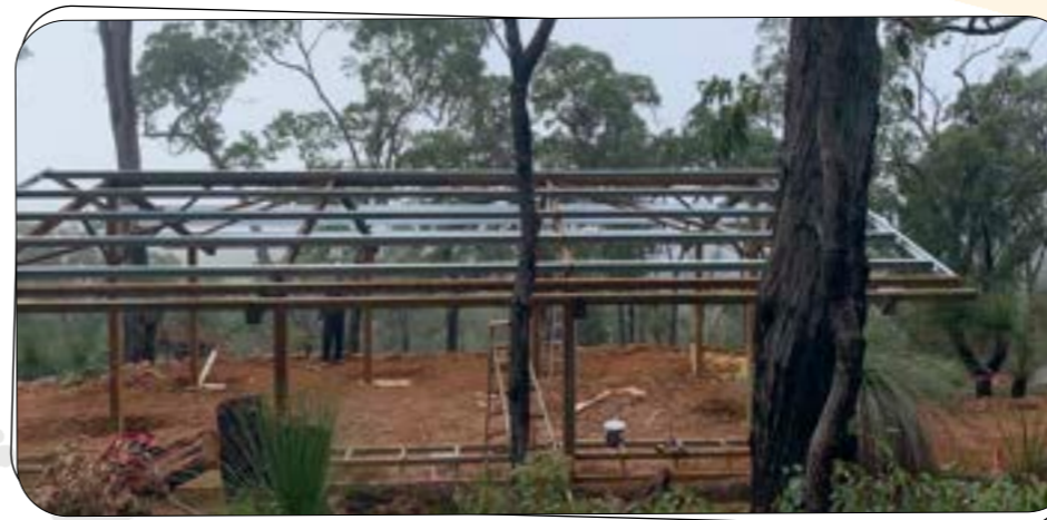
Construction of the shelter near Monadnocks is well underway.
