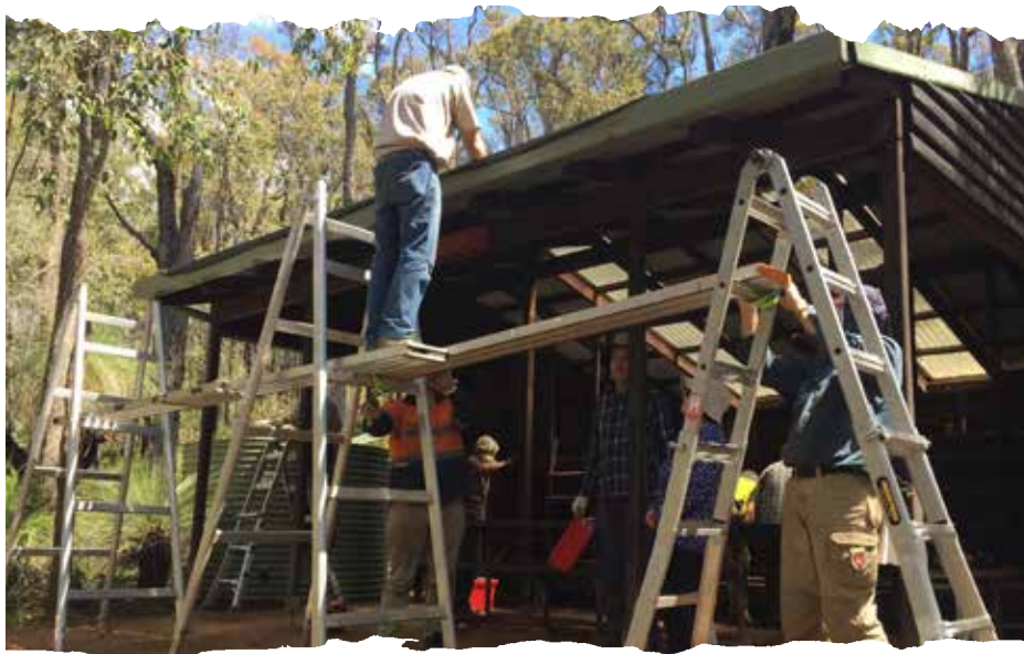
Trestles are used to reach the gutters at Noggerup Campsite
