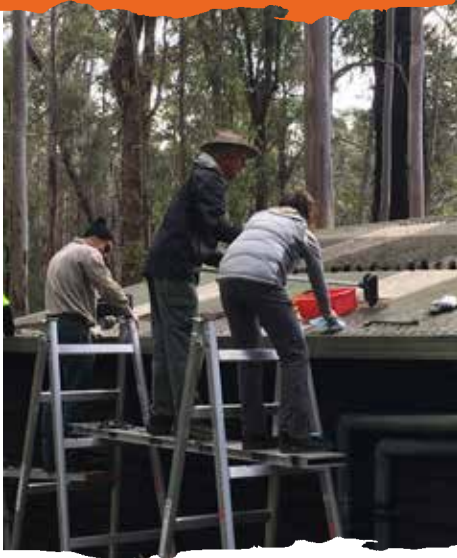
Volunteers replace gutter guard at Schafer Campsite
