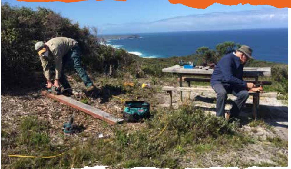
Not a bad work site! – at West Cape Howe Campsite
