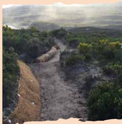
Newly stabilised track.
