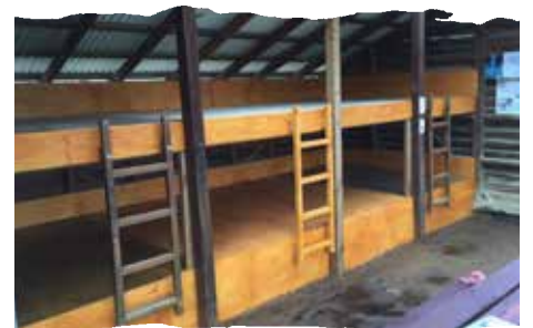
Additional bunk space built in where the table used to be.
