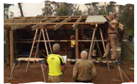
The shelter roof is extended.
