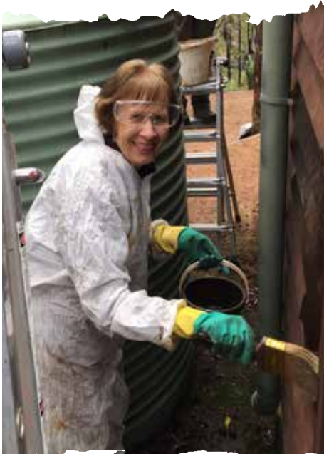
The cladding of Hewett's Hill shelter receives some fresh oil.
