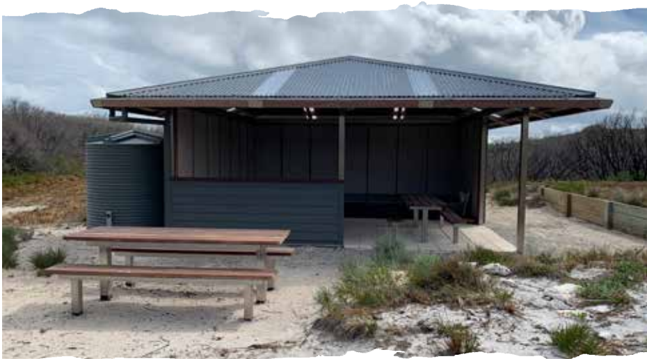
The new Sandpatch Campsite near Albany
