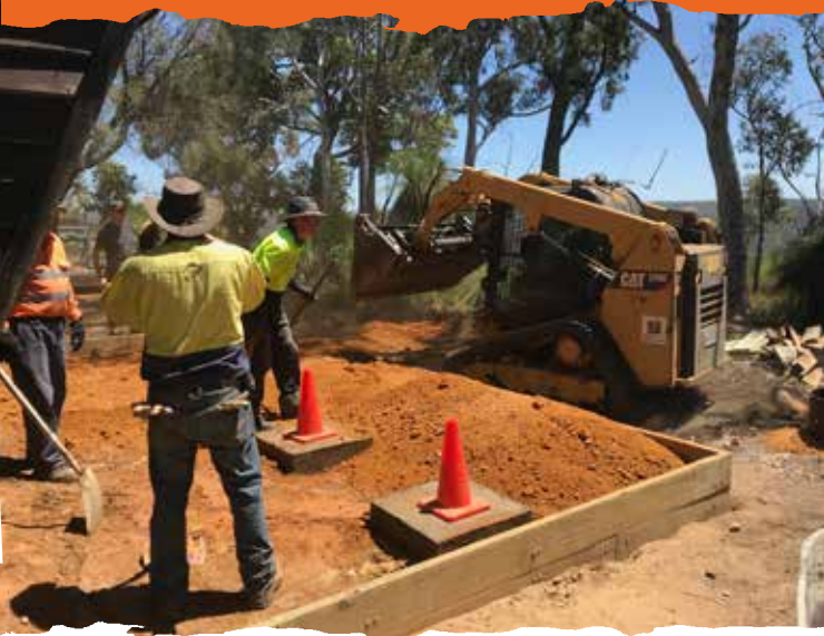
Waalegh extension earthworks
