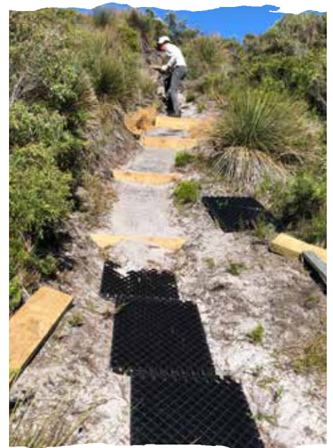
Erosion control methods include installation of timber box steps, 100% recycled polypropylene grids and coir mesh.
