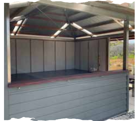
Due to Dieback restrictions, rammed earth could not be used at this site so the new shelter was built with fire-resistant fibre cement that looks like timber weatherboards. Let us know what you think.
