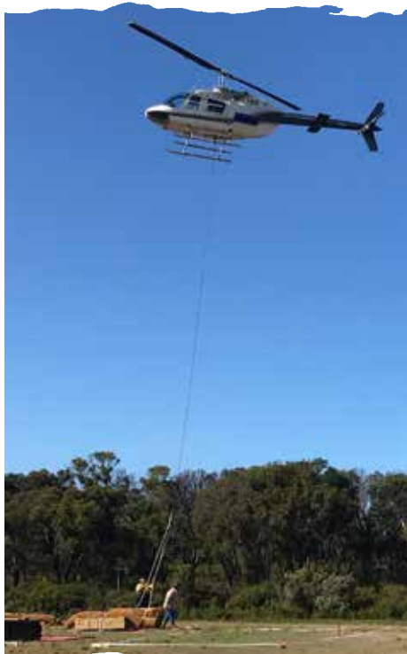
Four tonnes of materials and equipment were airlifted to remote sections of Track.
