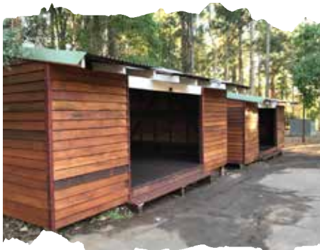
The rejuvenated shelters at Donnelly River Village
