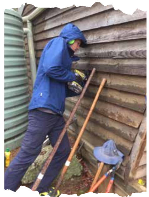
Fixing loose boards on Gringer Creek shelter
