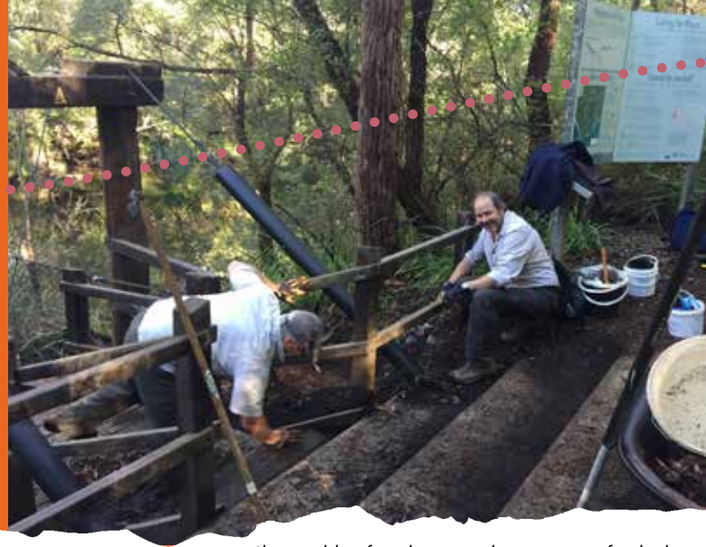
Clearing debris from the approach to Deep River foot bridge
