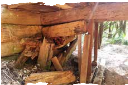
Several large timber members were replaced in the final stages of work on River Road Bridge.
