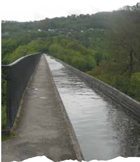
Telford's incredible aqueduct.
