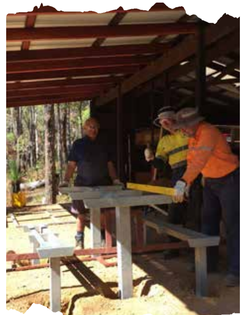
Installing tables at Swamp Oak Campsite
