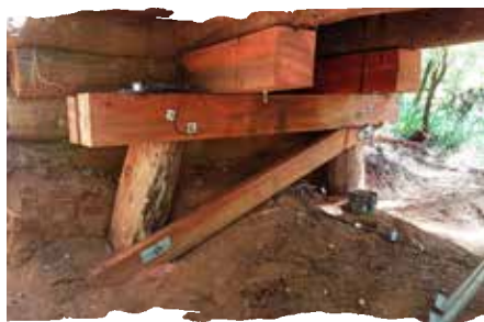
Several large timber members were replaced in the final stages of work on River Road Bridge.
