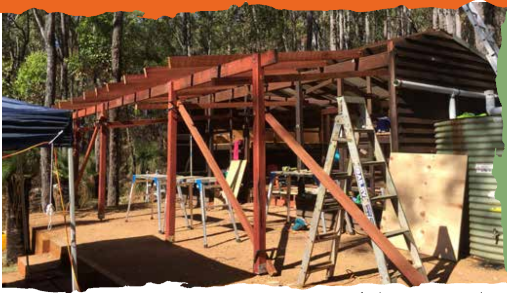
New roof and support structure erected
