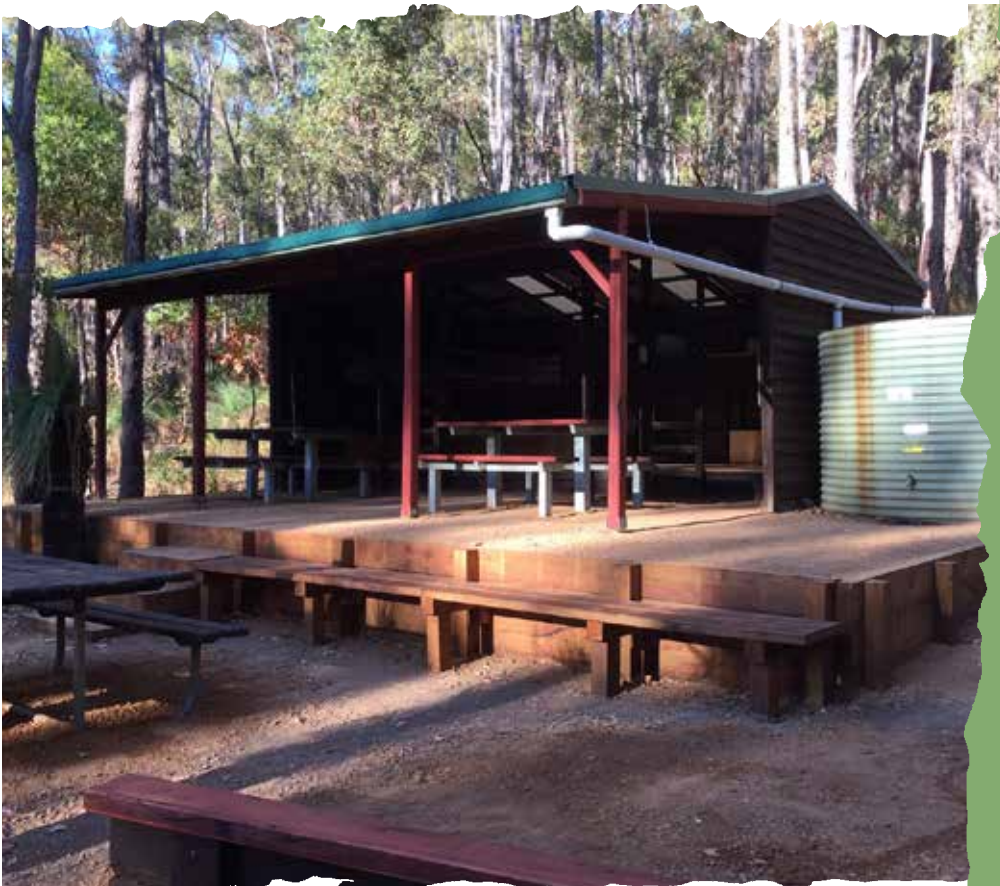
Swamp Oak Campsite extension completed
