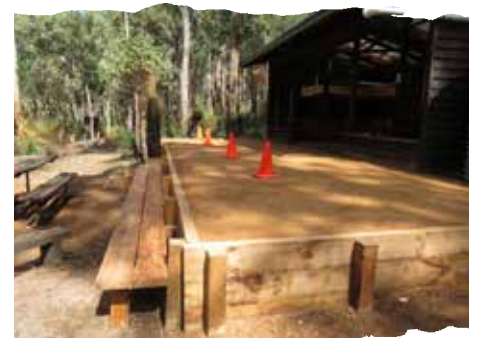
Completed retaining wall and floor.
