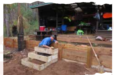
Tor Clarke installing steps
