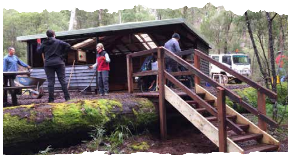
Spreading woodchips around the shelter and new stairs at Beedelup Campsite.
