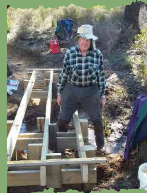
John Murphy installing his bridge.
