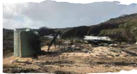
Any timber was reduced to ash and blown away.
