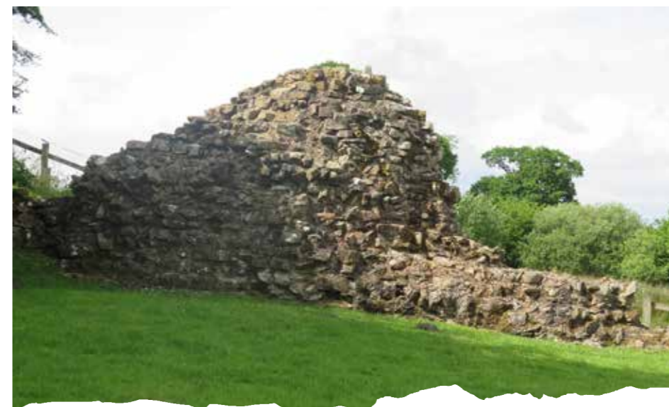
The Wall at Hare Hill
