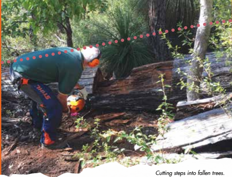
Cutting steps into fallen trees.
