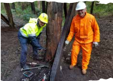
Replacing the brace bolt
