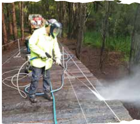
Cleaning the timbers with a high pressure hose
