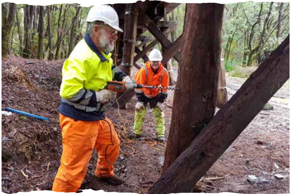
Drilling holes for the borate timber treatment application.
