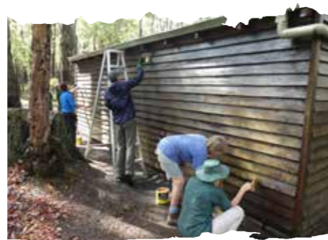
Re-oiling the shelter at Harris Dam Campsite
