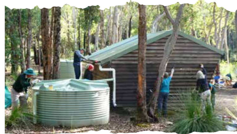
Cleaners, painters and oilers hard at work cleaning up the shelter at Ball Creek.
