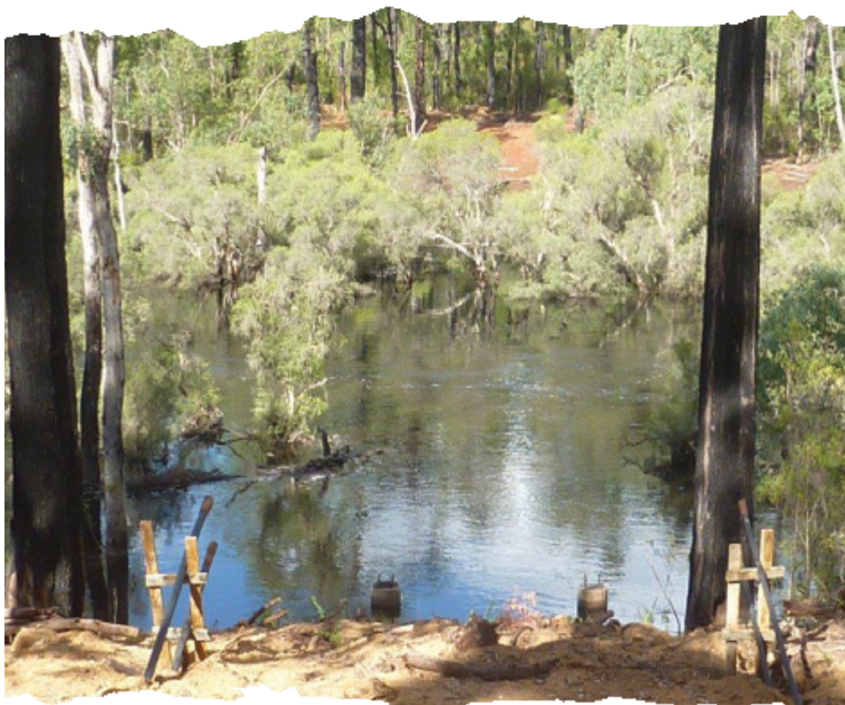
The new Murray River bridge footings submerged in flood.
