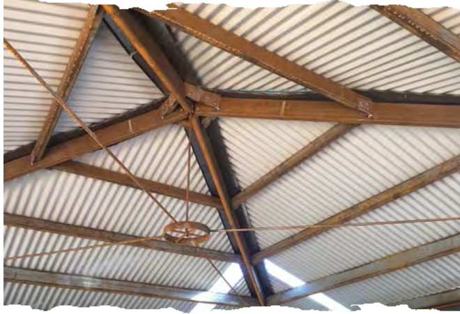
The weathering steel used throughout the campsite forms a stable rust-like appearance.
