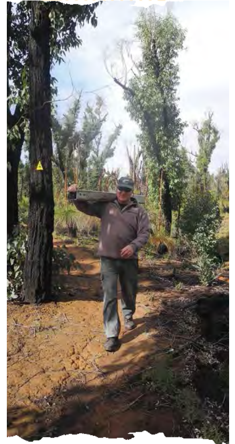
Rob Black and the other volunteers helped carry all the bridge components to the river bank ready for building.
