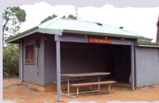
The new verandah looks as if it has always been there.
