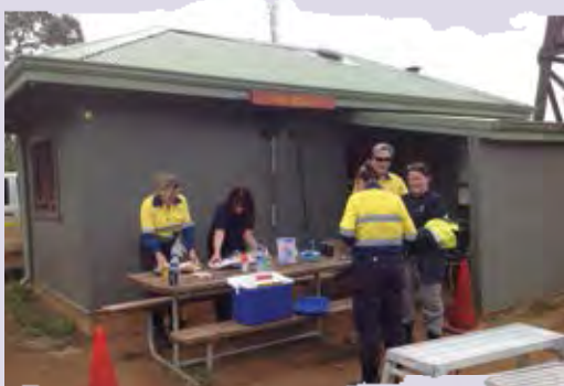
Alcoa volunteers before starting work on the new verandah.
