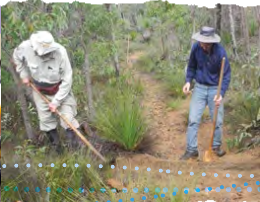
Volunteers John Murphy and Rob Willis-Jones installing water bars.
