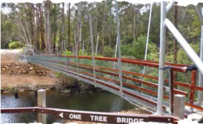
The new suspension bridge at One Tree Bridge provides safe passage over the Donnelly River for Bibb Track walkers, and cyclists on the Munda Biddi Trail.
