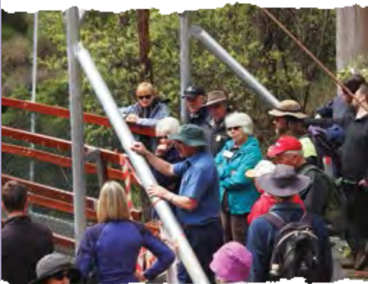
Parks and Wildlife officer, John McKenzie, describes the process of constructing the new bridge.
