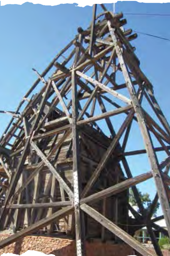
Sons of Gwalia mine headframe, constructed in Oregon in 1899.
