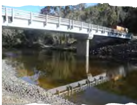
New Southampton Bridge
