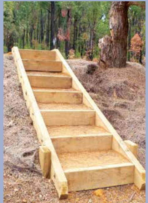
New steps installed near the conveyor belt in the Wellington District.
