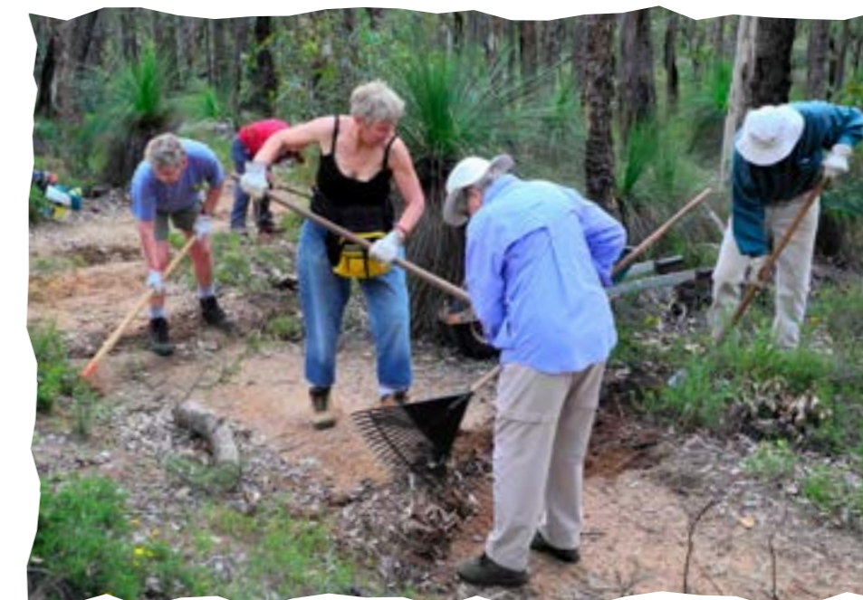
Installing water bars in the Perth Hills.
