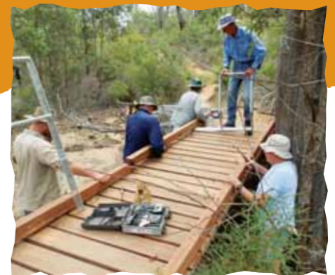
Fitting railings to bridge erected in March 2011 by volunteers.
