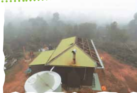
Roof restoration in progress
