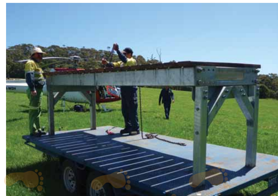
A complete kit bridge, ready for installation, was flown into Long Point to replace an old single plank bridge which had become unsafe. Use of the helicopter saved DEC staff and volunteers from having to carry the bridge piece by piece for 3.5 kilometres.
