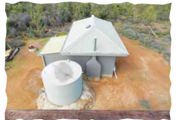
The completed upgrade
