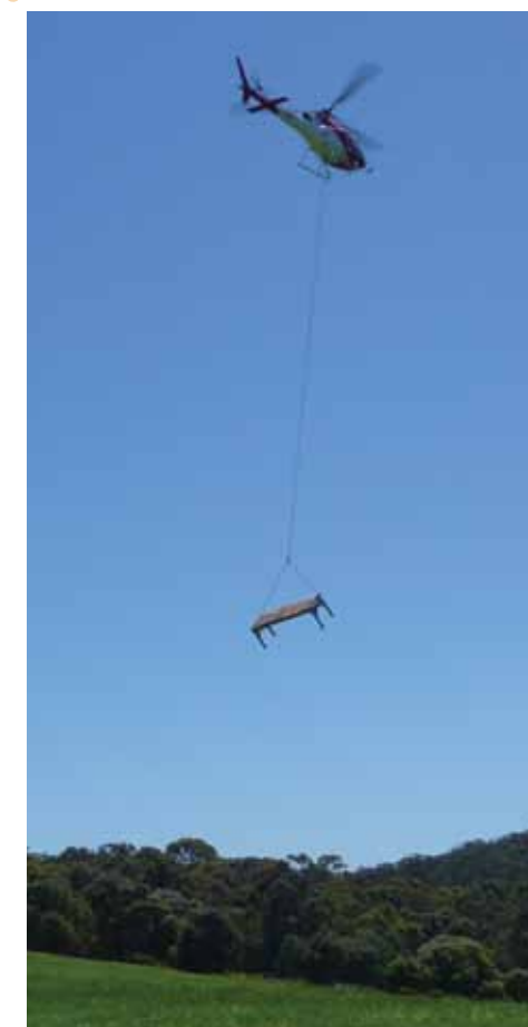
A complete kit bridge, ready for installation, was flown into Long Point to replace an old single plank bridge which had become unsafe. Use of the helicopter saved DEC staff and volunteers from having to carry the bridge piece by piece for 3.5 kilometres.
