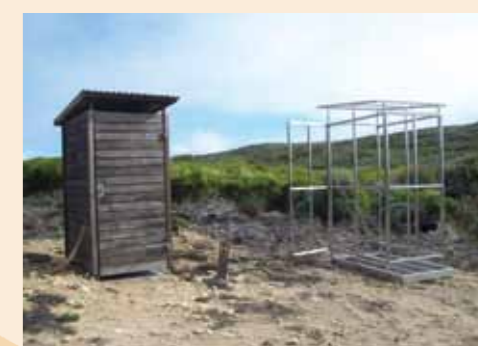
Stainless steel is used for the new toilet frames
