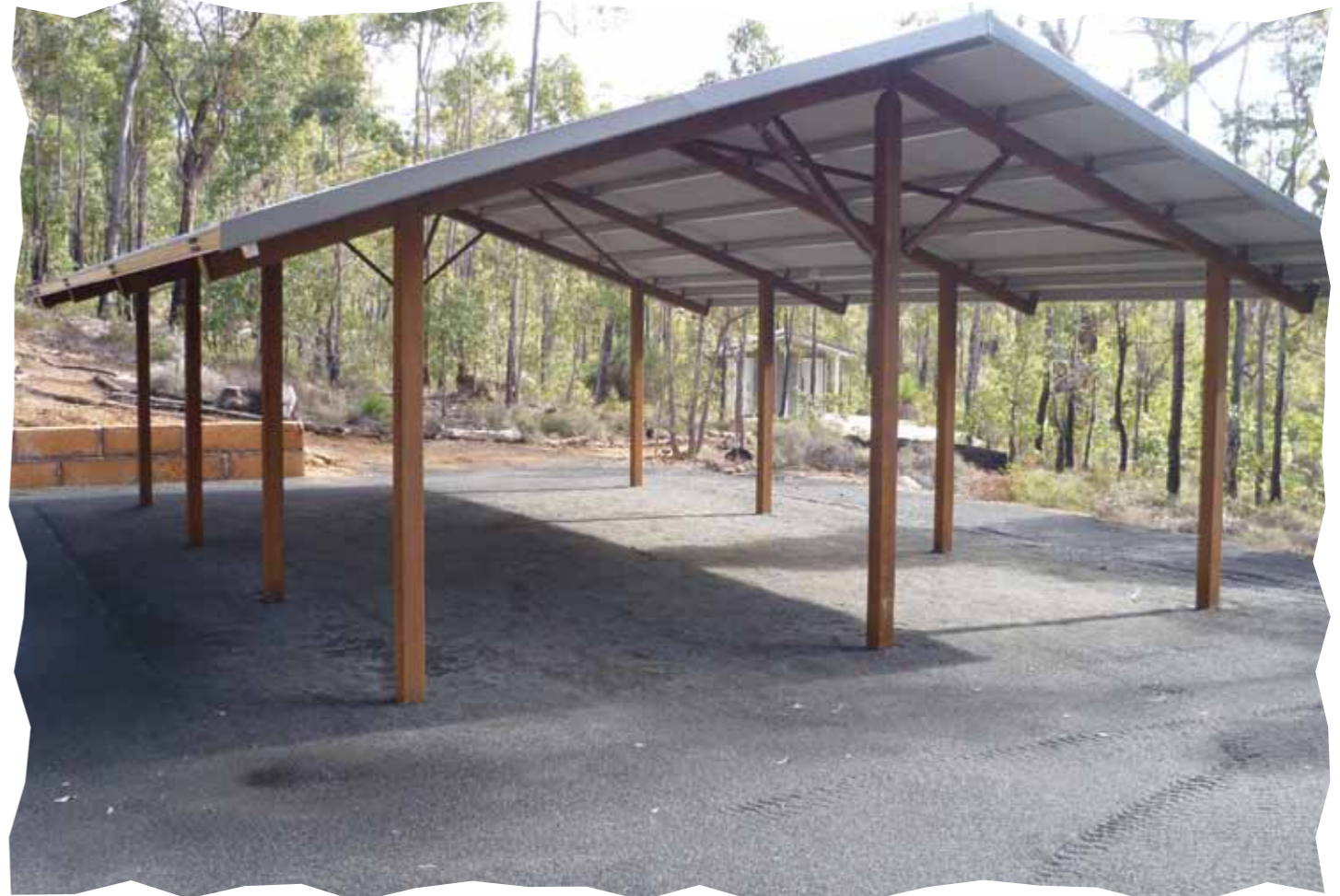
Cooking shelter at the new Lyalls Mill campsite near Yabberup
