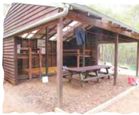
Tom Road shelter after refurbishment
