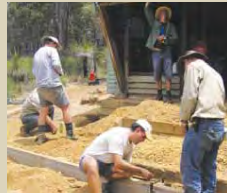
Work on the terracing in front of the shelter
