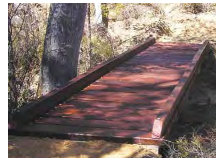
The finished product. Wood has been oiled, and the approach trails built.
