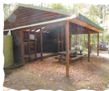
Tom Road shelter before refurbishment
