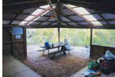
View from inside Bibb shelter
