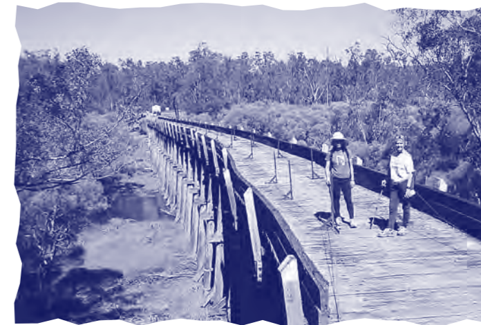
Long Gully Bridge
