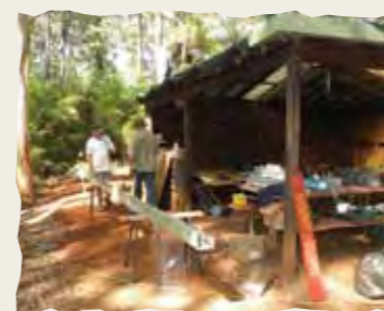
Replacing the guttering
