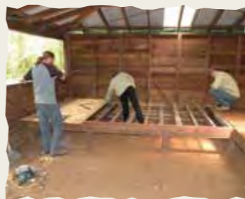
Replacing the old platform with marine ply
