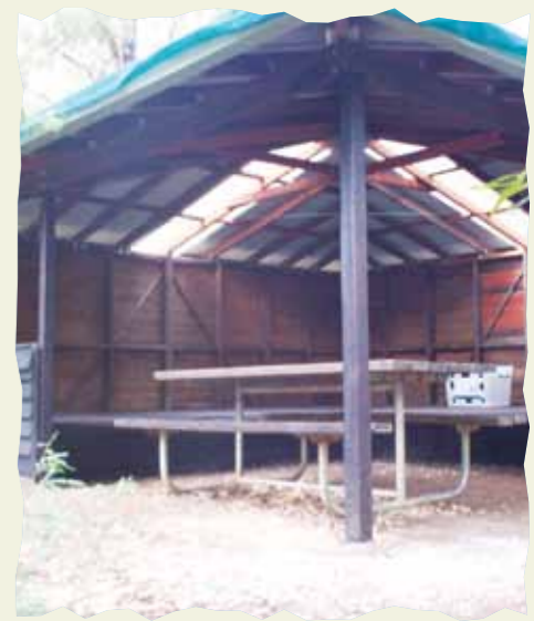
The rebuilt shelter is now open to walkers
