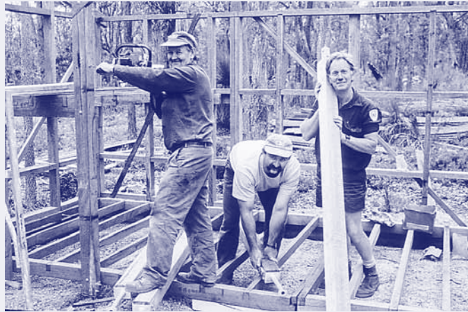
Then - CALM crew constructing Beraking Campsite
