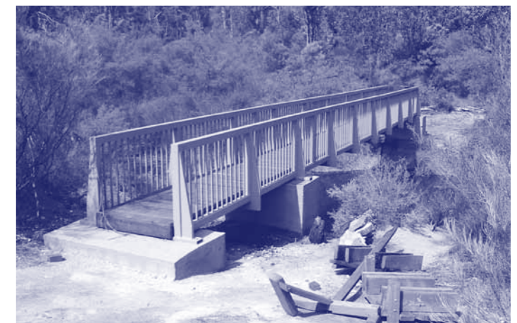
Canning Bridge just prior to completion
