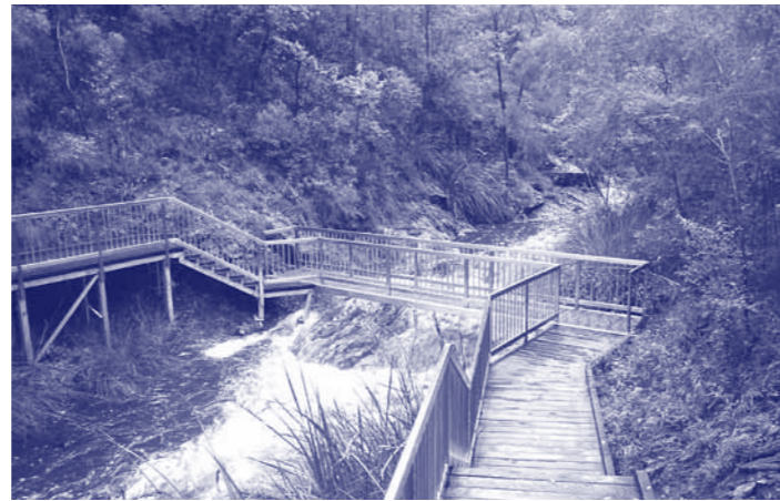
New bridge at Beedelup Falls
