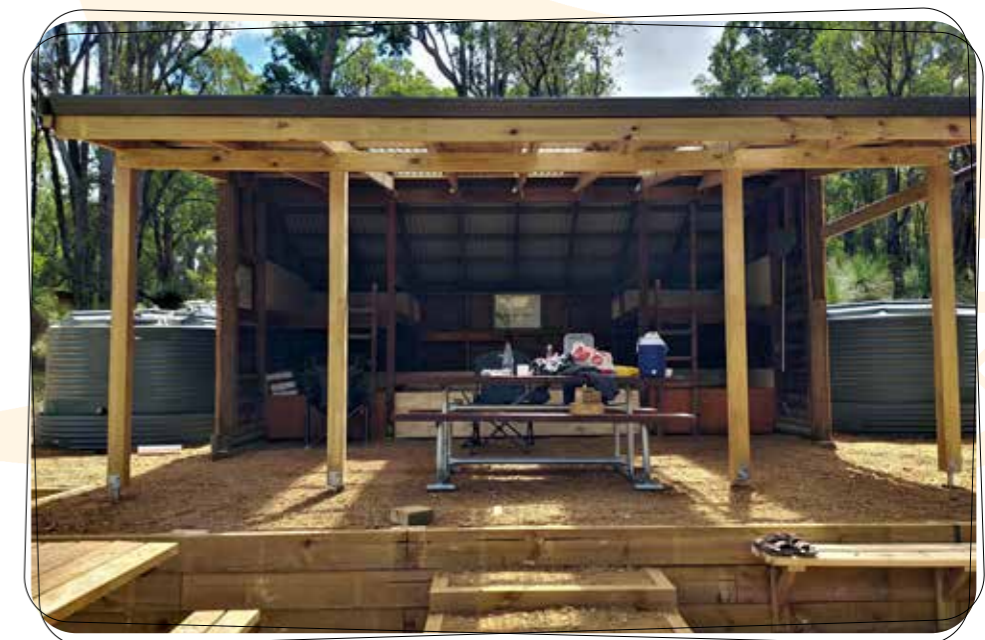
The extended shelters include two water tanks and more seating.
