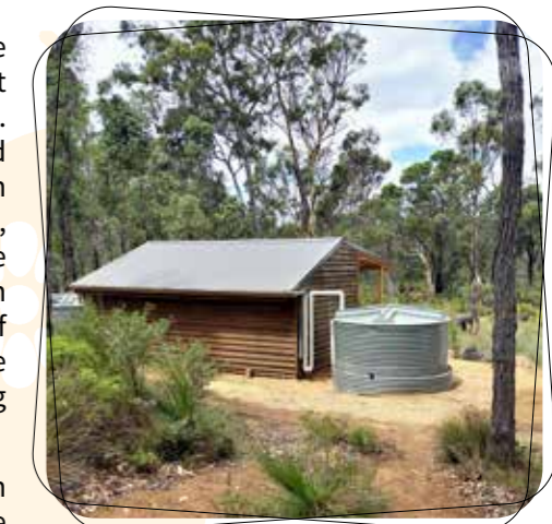
The new roof at Gringer Creek Campsite is in woodland grey.
