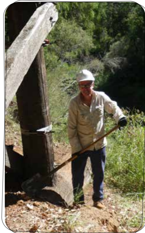
Nigel working at River Road Bridge.
