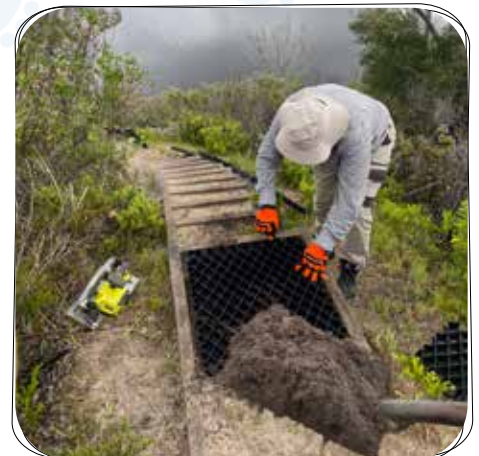
Track pad installation - Irwin inlet
