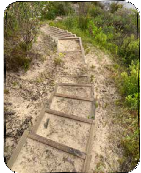
Steps at Irwin Inlet before track pad installed.
