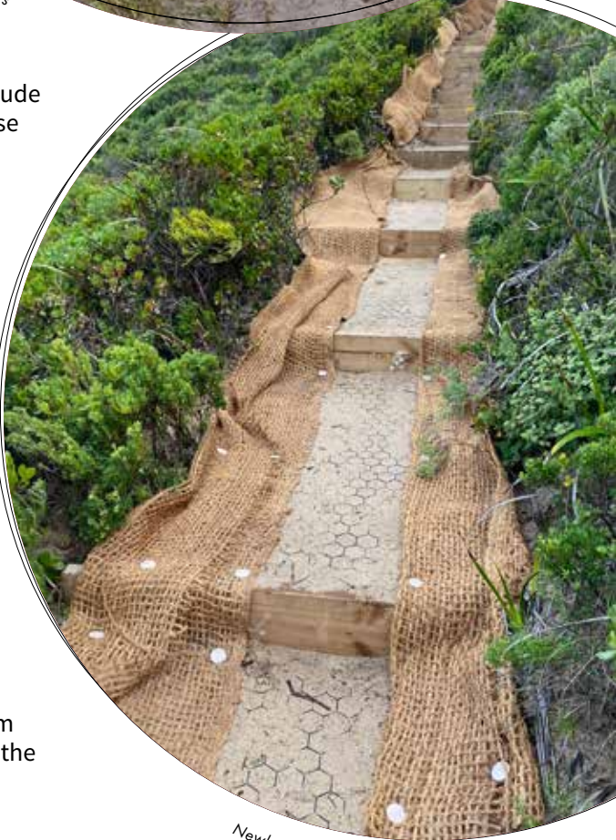
Newly laid track pad & coir mesh
