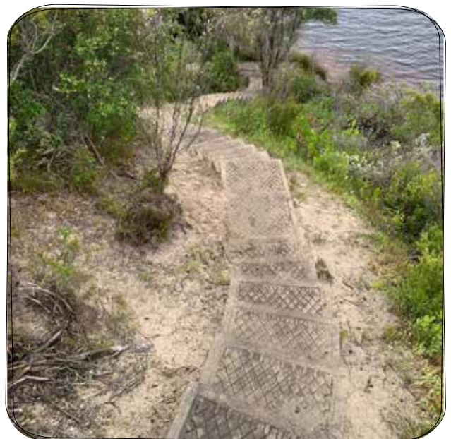
Steps at Irwin inlet after remediation.
