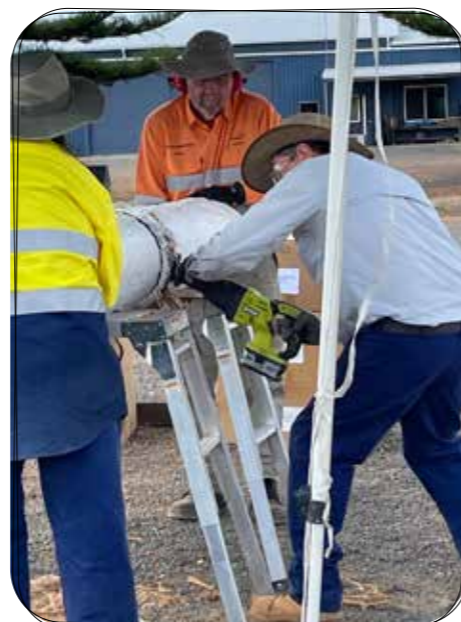
Cutting coir matting for remediation work.
